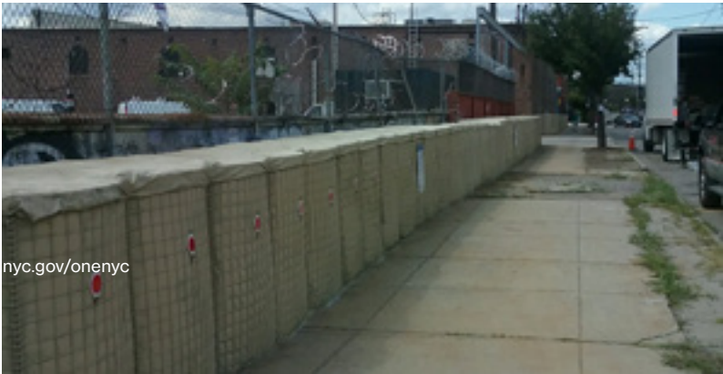
Hesco barriers deployed along Beard Street as part of the Interim Flood Protection Measures program mitigate low-level flooding in Red Hook.
