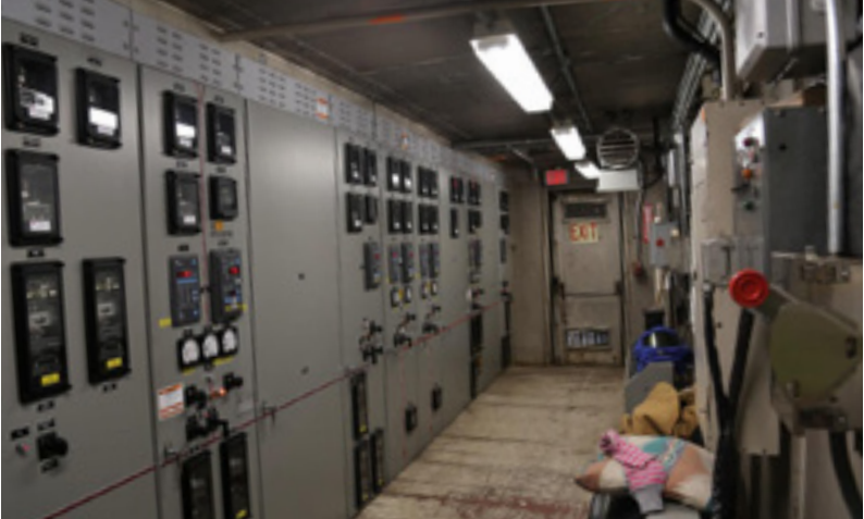
As part of broader resiliency upgrades at the Bowery Bay Wastewater Treatment Plant, DEP will seal and protect this switchgear room with a flooding barrier.
